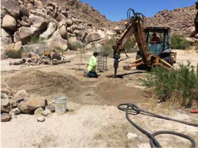
PREP WORK FOR SHELTER INSTALL
